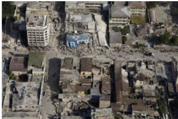
Some collapsed buildings after Haiti earthquake. Puerto Príncipe. 2010. Source: Wikipedia.
